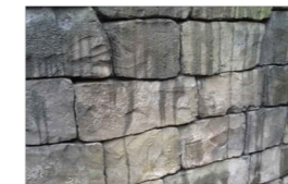
IMAGE REFERENCE Q.005 (QUEUE LINE WALLS)
