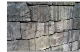
IMAGE REFERENCE Q.005 (QUEUE LINE WALLS)
