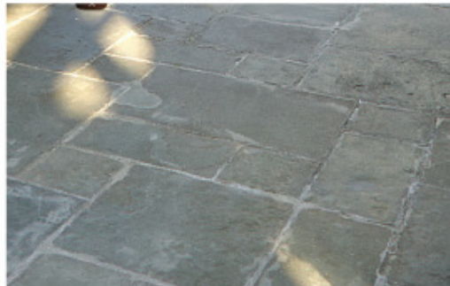
06. Church-style floor stone slabs. - Pattern impressed concrete to mimic similar effect
