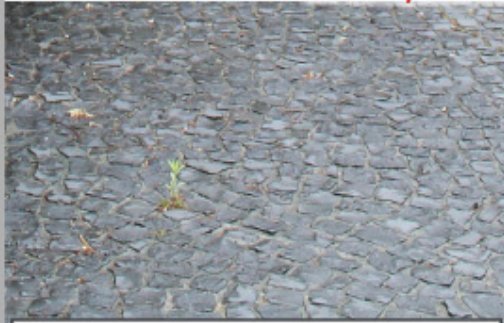
02. Cobbled stones to match / complement existing on site
