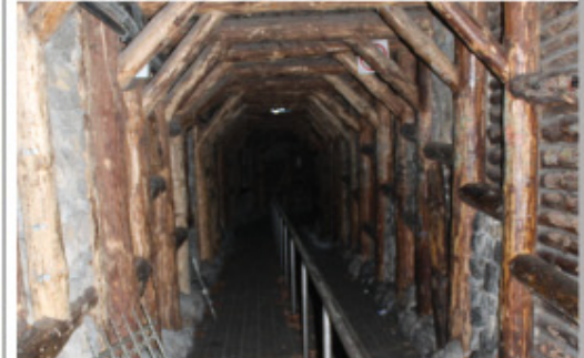
10. Timber half-round panelling and beams (existing within qine tunnels)
