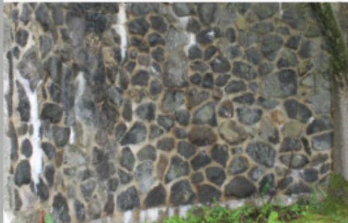
03. Irregular stone wall construction
